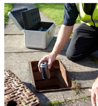
Attaching a data logger to a valve.
