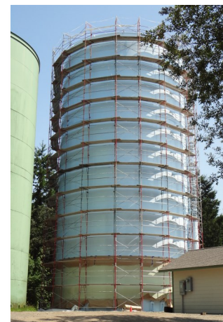
Construction on the Tanglewilde-Thompson Place reservoir in 2012.
