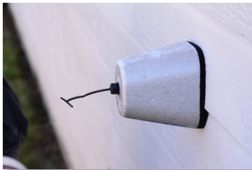
A faucet cover installed on an exterior faucet.
