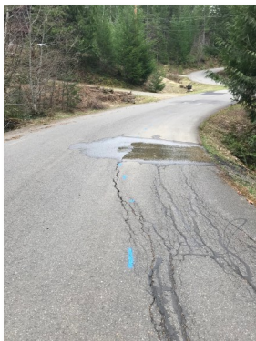
A large puddle on a dry road, caused by a mainline leak.
