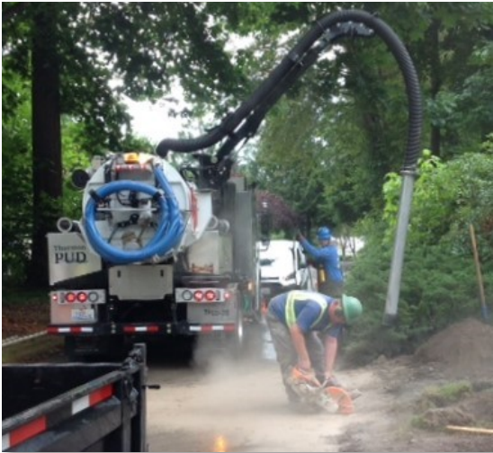
A PUD crew working to repair a water leak, classified as a repair. Taken in 2018.
