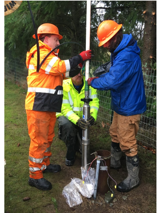
New well pump installation at the Post Lane water system.
