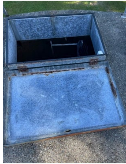
Reservoir #1 intact hatch seal.
