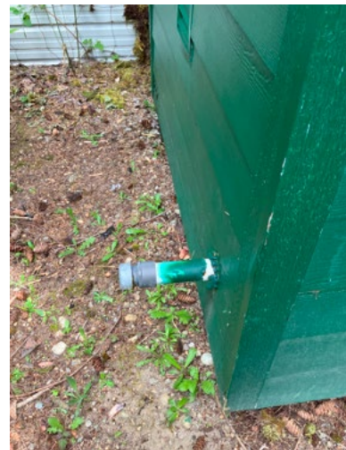
Capped off pipe at the pump house, can be used for flushing.
