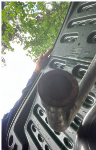
S01 well vent intact.
