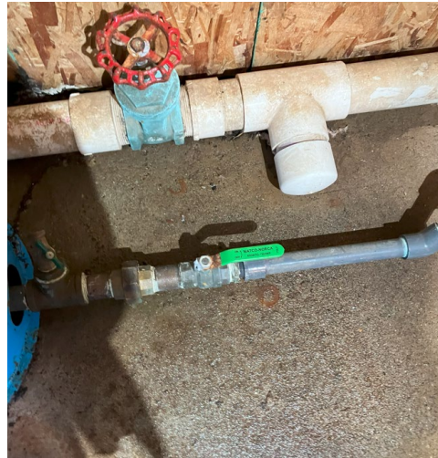
Bladder tank's isolation valve, no PRV.
