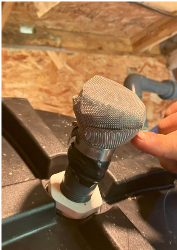
Reservoir #2's screened vent.
