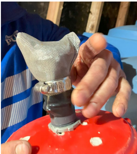
Reservoir #1's screened vent.
