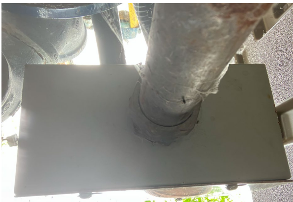
S01 junction box, conduit sealed.
