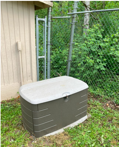
Rubbermaid enclosure for S01 well head.
