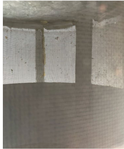
Reservoir #2 intact vent screen.
