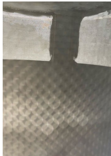
Reservoir #1 intact vent screen.
