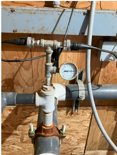
Pressure gauge at booster pump discharge.
