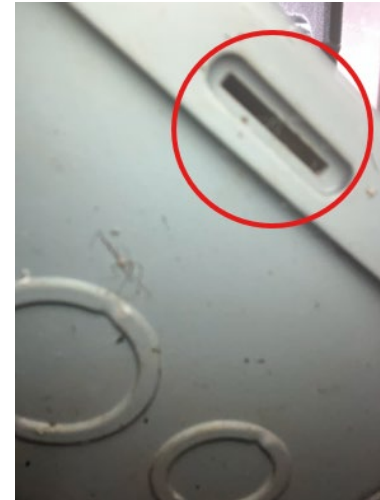
S01 junction box, with an opening.
