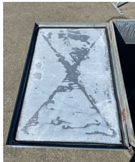
Reservoir #2 intact hatch seal.
