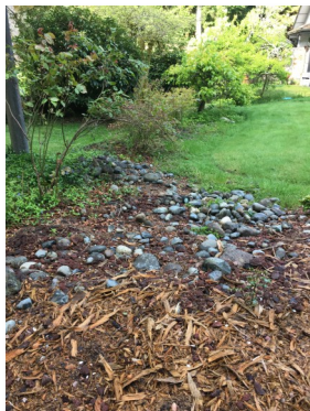
There's a meter buried under there!
